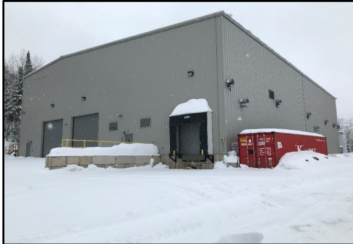
Water Treatment Plant Expansion, 2020.
