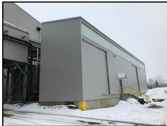
Three-sided enclosure surrounding the thickeners, 2019
