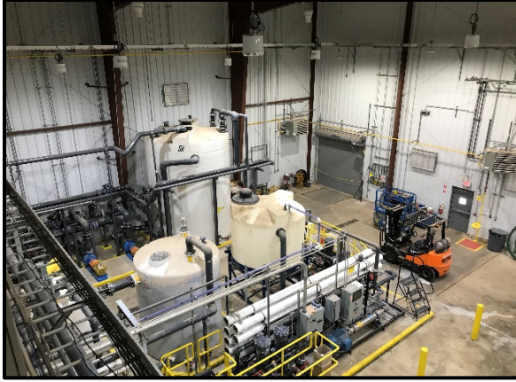
Interior of the new WTP expansion including installed equipment for the concentrator RO and clarifier, 2020.
