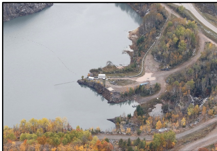
Aerial view of tailings lines and shore vault at HTDF, October 2018
