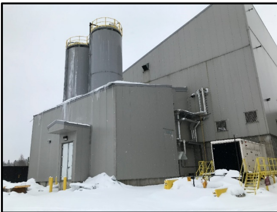
Enclosure around the lime and soda ash facility, 2019
