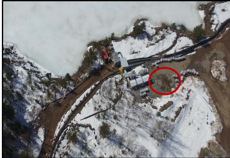
Mill WTP Fenton Reactor Area - Location of Spill, March 2019
