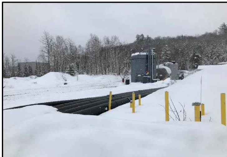
Location of MW-701 well cluster relative to the sulfuric acid spill location.
