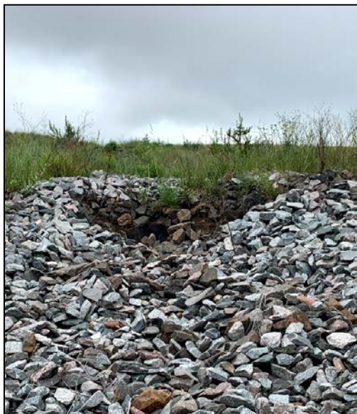
NCWIB #3 – Before riprap repairs
