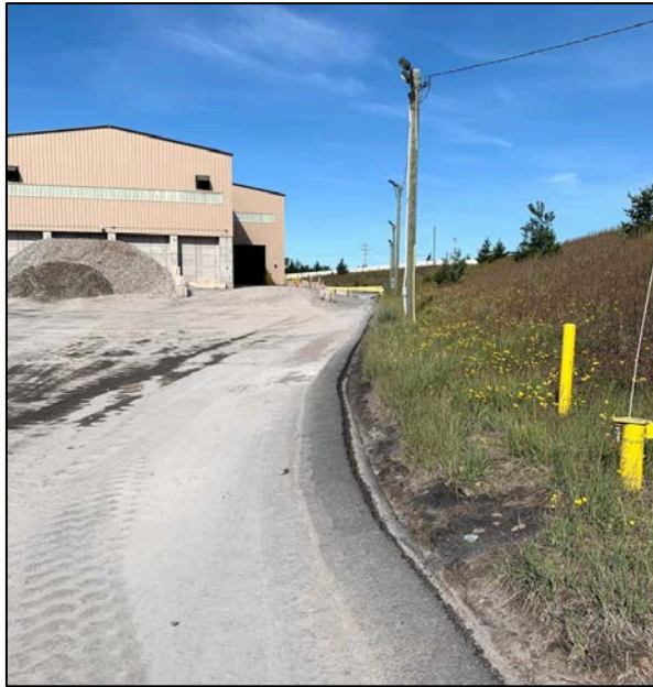
New curbing located near QAL067A
