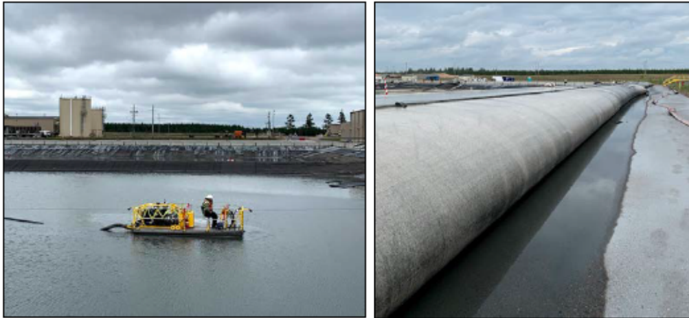
Dredge On the Basin and Full Geotube, May 2021
