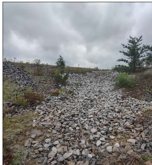
NCWIB #3 – After riprap repairs
