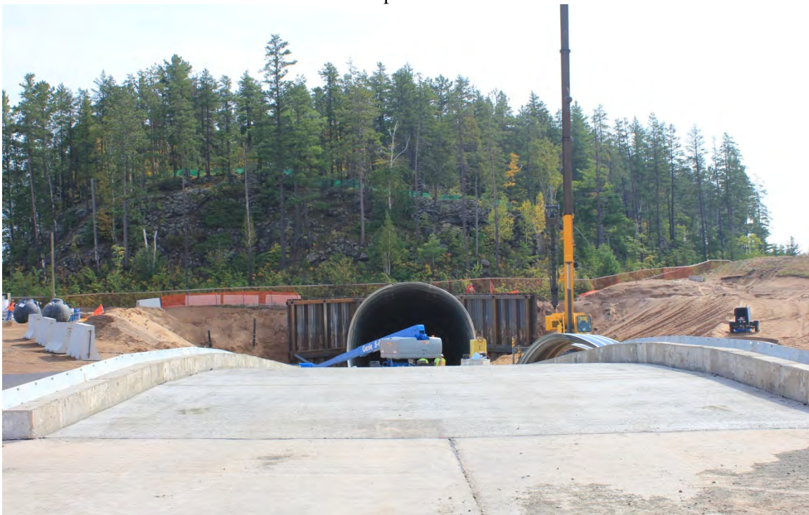
Portal Construction, August 2011
