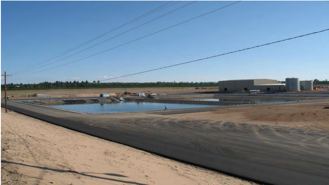
Contact Area Paving Underway, August 2011
