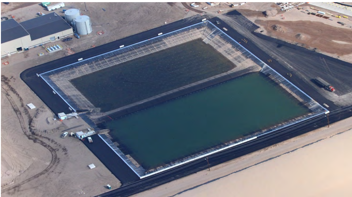
Contact Water Basins, September 2011
