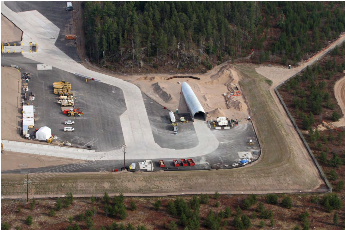
Steel Arch Complete, 2011
